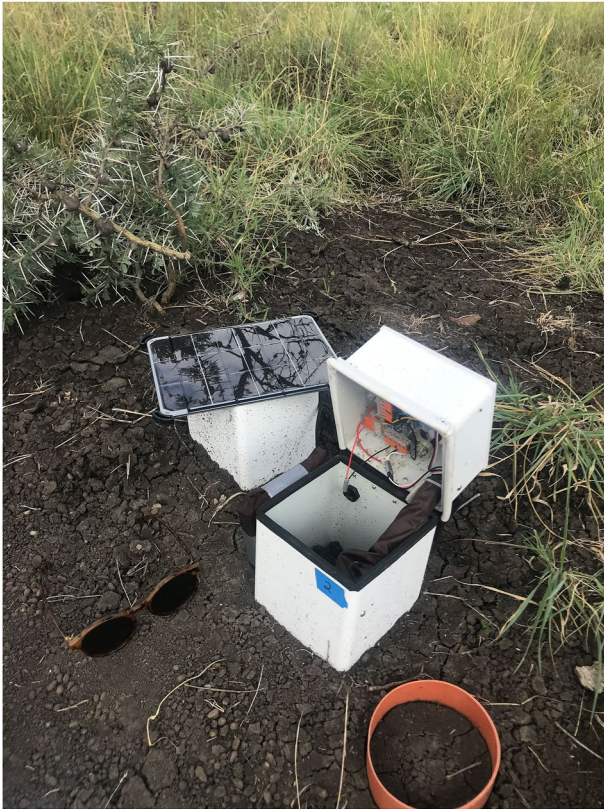
Figure 3. A fluxbot installed in the field, in its open position, with actuator fully extended. Collar for manual data collection at bottom right.
