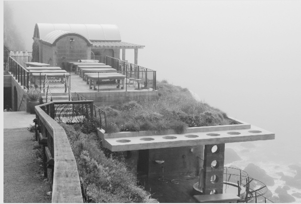
FIGURE 21.3. Green roof on bath house at Esalen Institute, Big Sur, California. Photograph by Paul Kephart.
