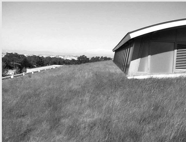
FIGURE 21.5. Coastal terrace grasses on roof at Gap headquarters, San Bruno, California. Photograph by Paul Kephart.
