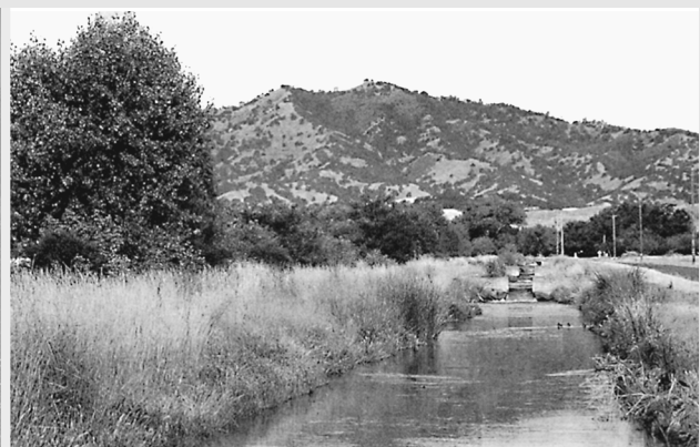
FIGURE 21.7. Irrigation ditch planted with native grasses for wildlife, soil stabilization, and reduced annual maintenance costs. Photograph by John Anderson.
